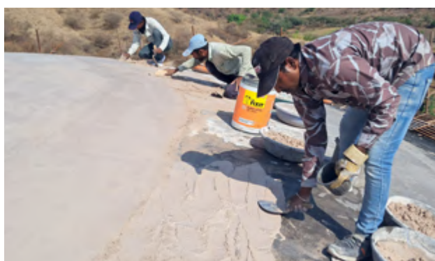
Applying the lime plaster
