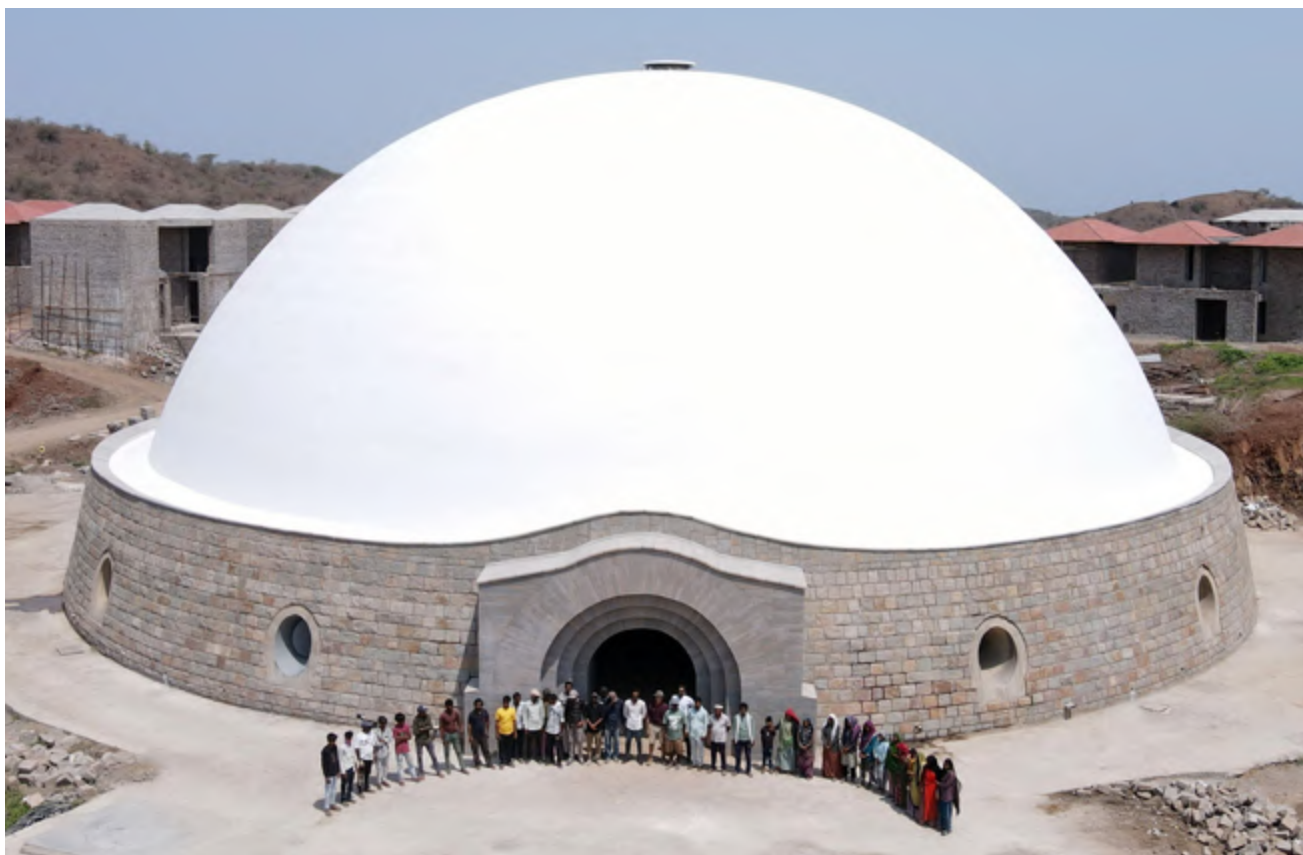
Dome waterproofed in 6.5 weeks
