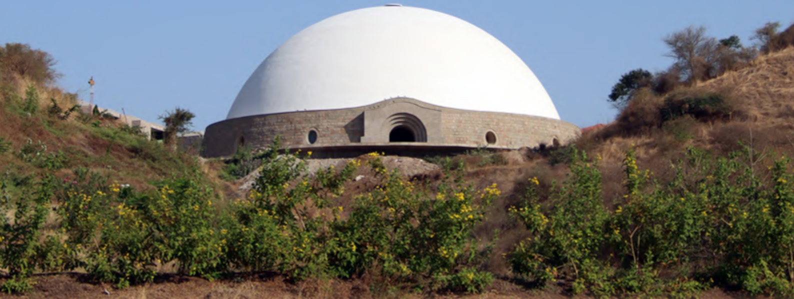
The largest CSEB Dome is now wrapped with waterproofing layers
