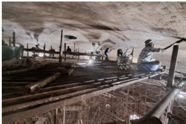
Finishing inside of the dome
