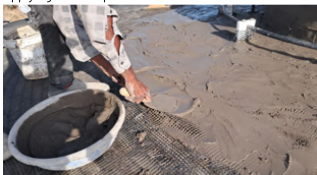
Ferrocement layer with 2 coats of fibre mesh
