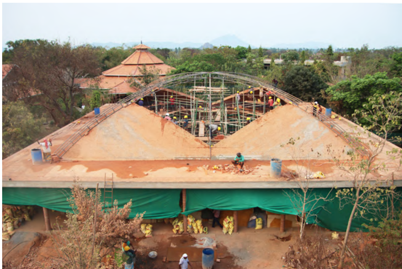
Squinches of the dome before dismantling
