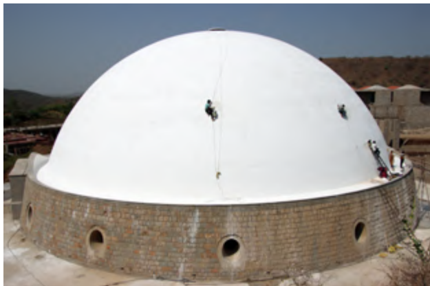
5th week: Applying the lime milk to fill the micro cracks
