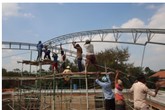
Assembling the template on the diagonals
