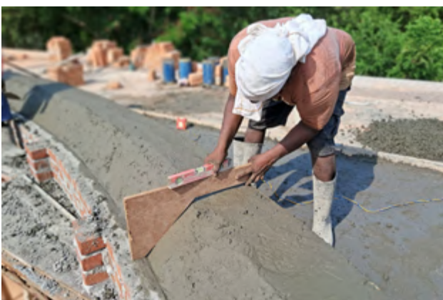
Circular slab & springer beam casting
