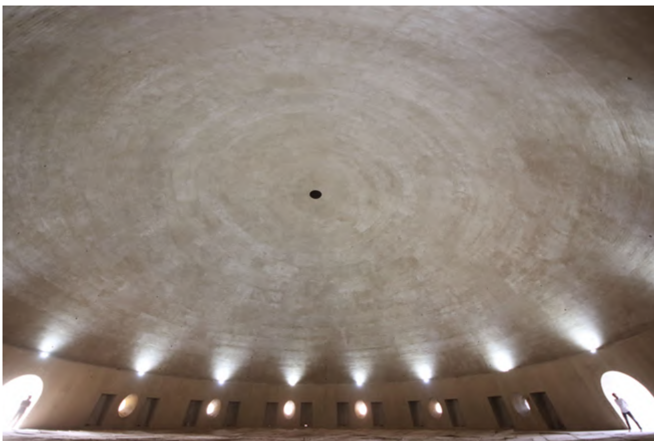
Finished surface of the inside of the dome
