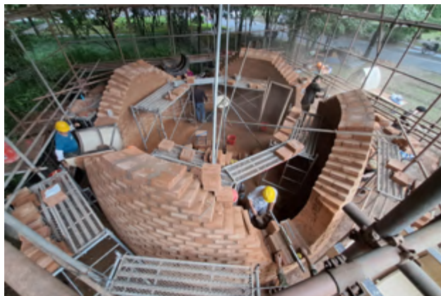
Pointed dome construction integrating circular windows
