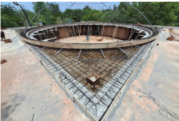
Extended slab reinforcement
