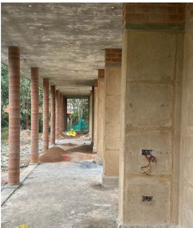
Corridor with PEC walls & composite columns in view
