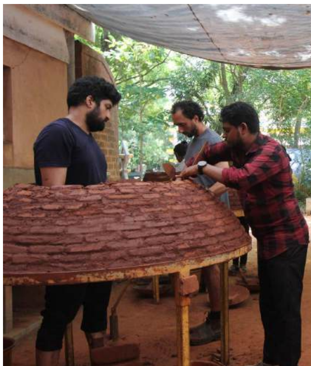
Participants working on a segmental dome with CSEBs
