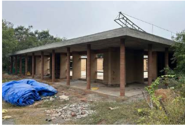
Hall ready to be crowned with a cloister dome
