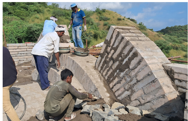
Tympan arches under construction
