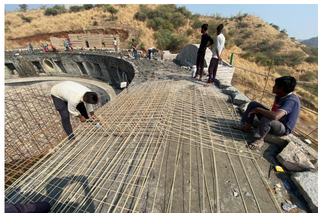
Glass Fiber Reinforced Polymer (GFRP) bars for ring beam
