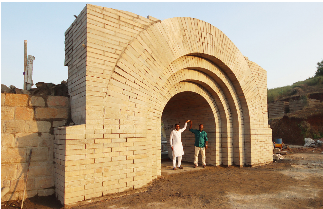
First entrance vault and its tympan arches completed in 11 days
