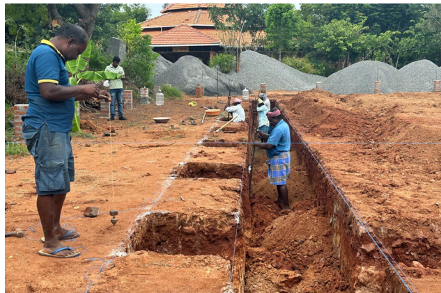
Foundation excavation of inner walls and buttresses.
