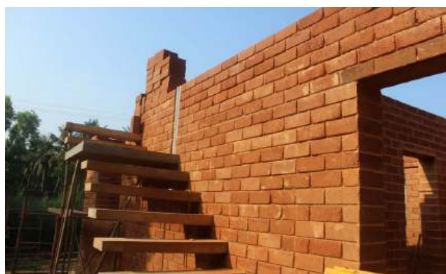
Building the external staircase to the terrace
