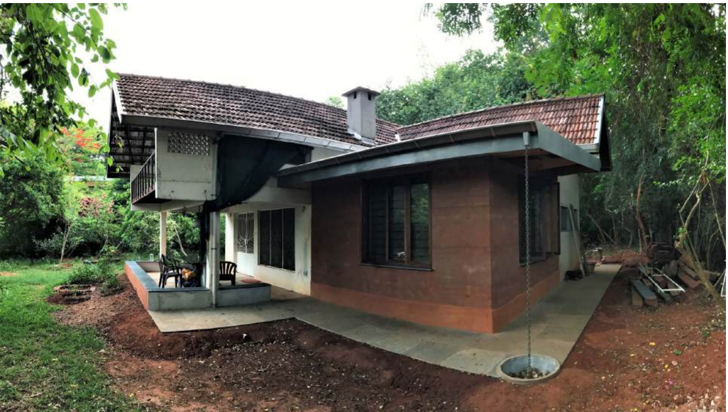
Top: Starting the bedroom addition in Utilité Community in Auroville Bottom: The completed cement-stabilized rammed earth bedroom addition
