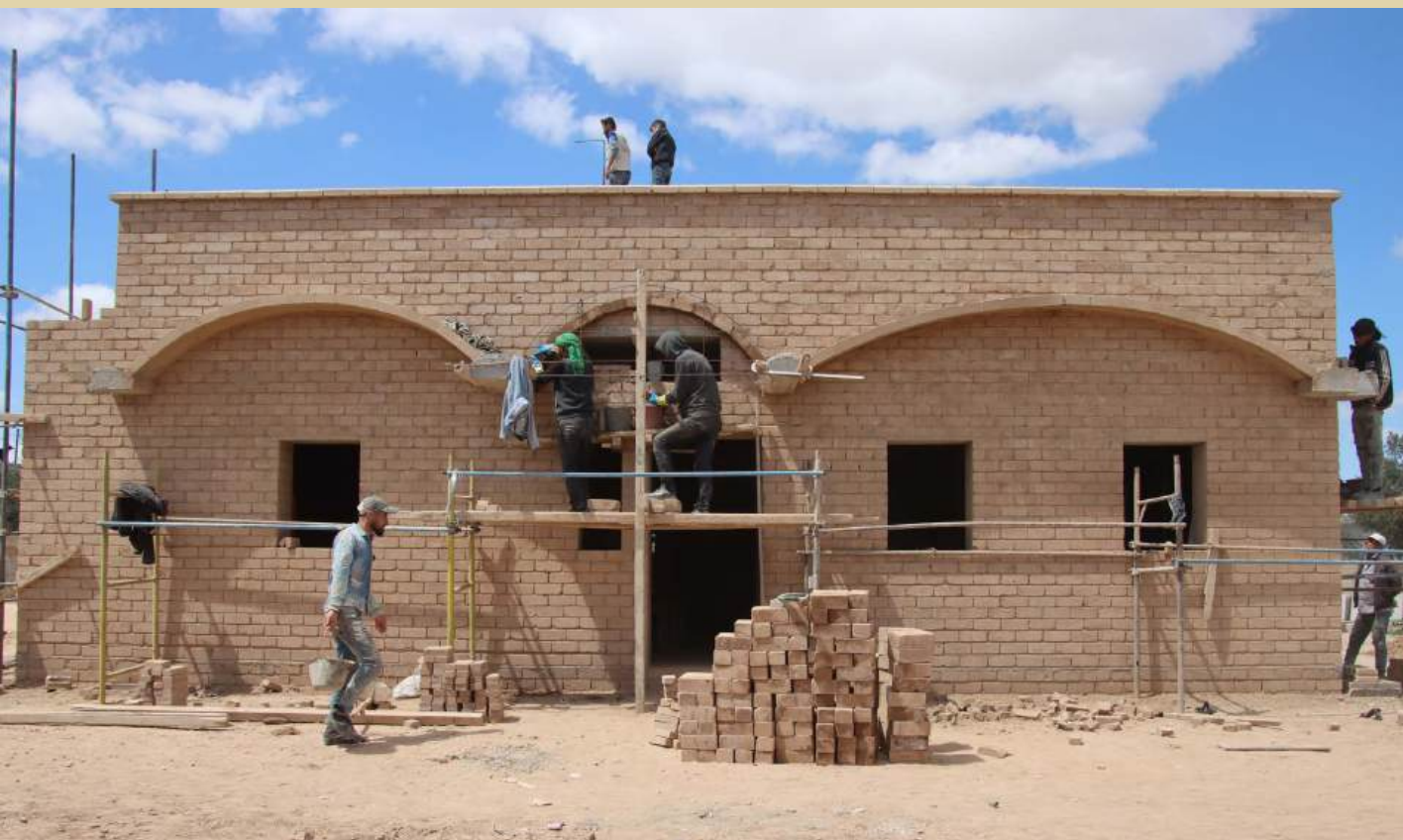
Construction of the overhangs on the Barri Demonstration House
