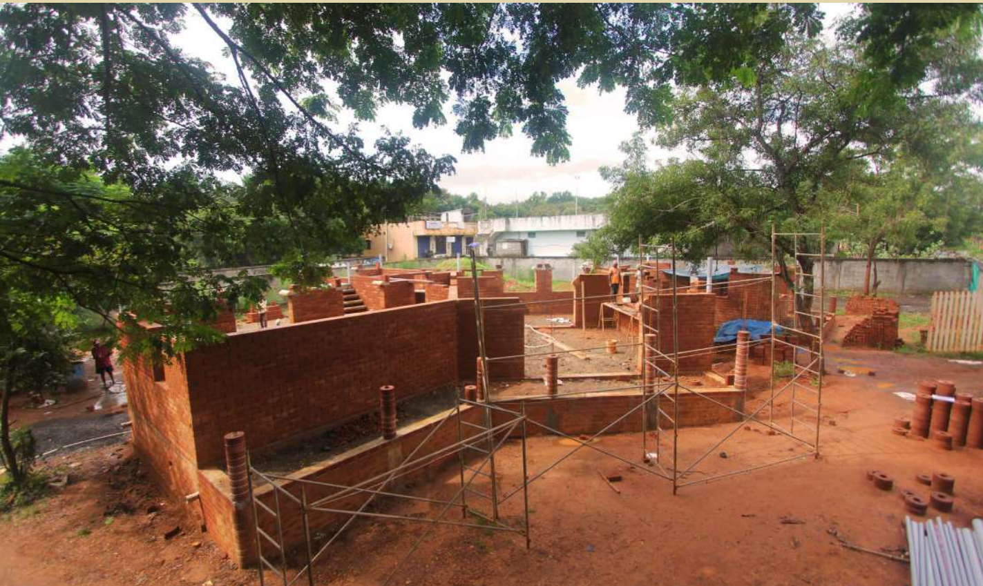
Construction of the Bonnet Family Residence
