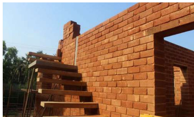
Building the external staircase to the terrace
