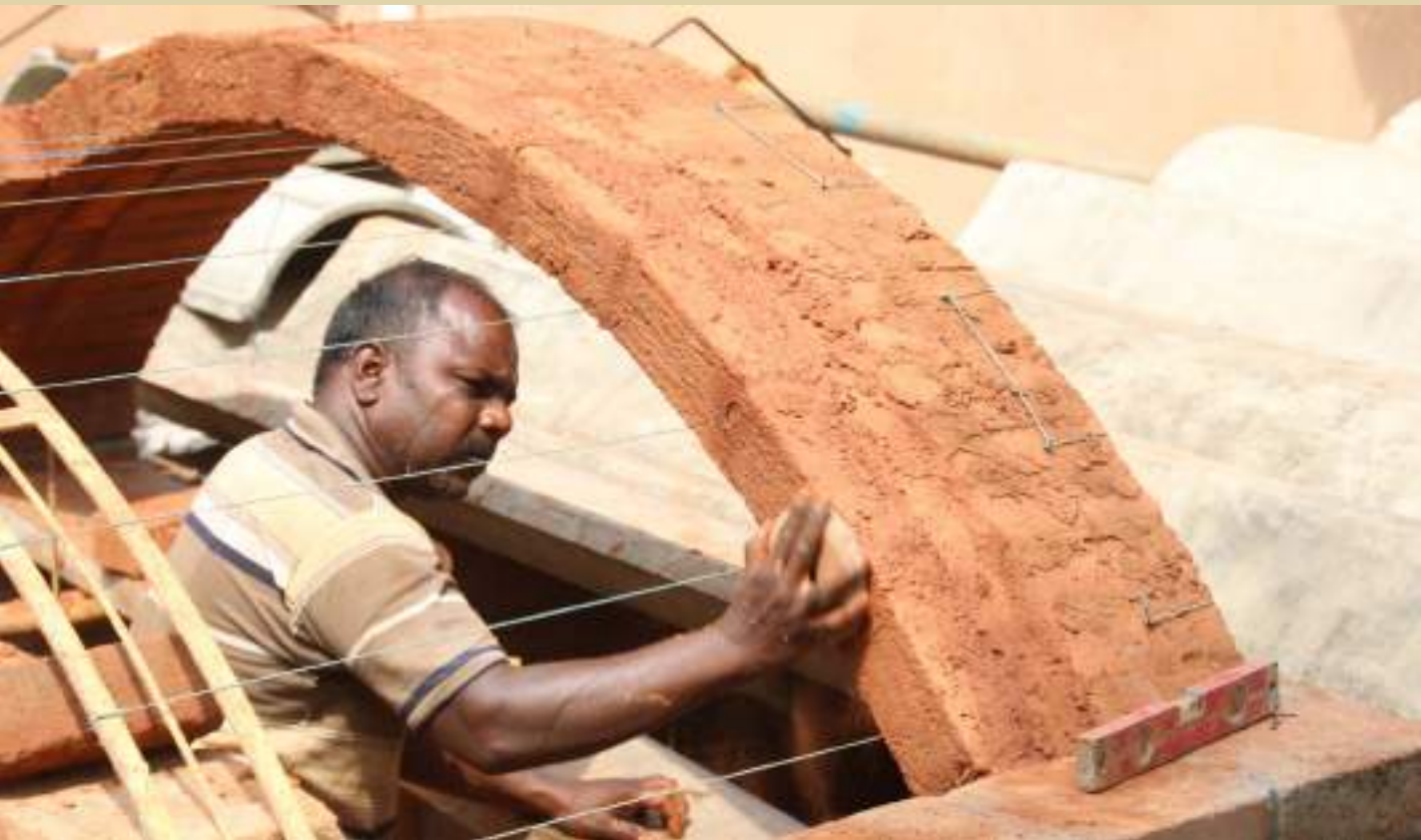
Mason Mani working on the adobe vault
