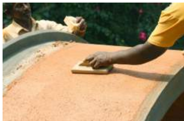
Applying the lime-based waterproofing
