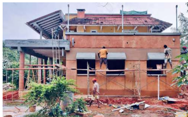
Construction on the Petite Ferme house extension
