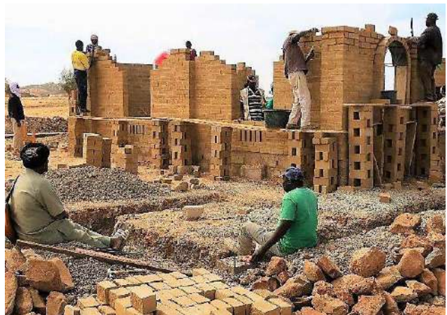
Construction practices in Mauritania (© ETR-ML)
