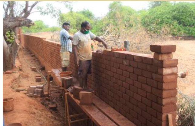
AVEI masons working on the compound wall at Aureka
