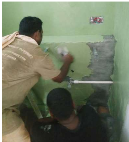
From top to bottom: mixing the green tadelakt, applying the plaster on the shower and bathroom walls, rubbing in black soap with the stone, the tadelakt walls with matching oxide flooring drying, and a detail of the tadelakt in the shower
