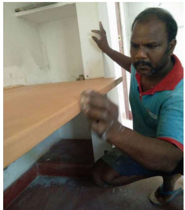
Mani applying the earth tone tadelakt mix and compressing the tadelakt with the stone
