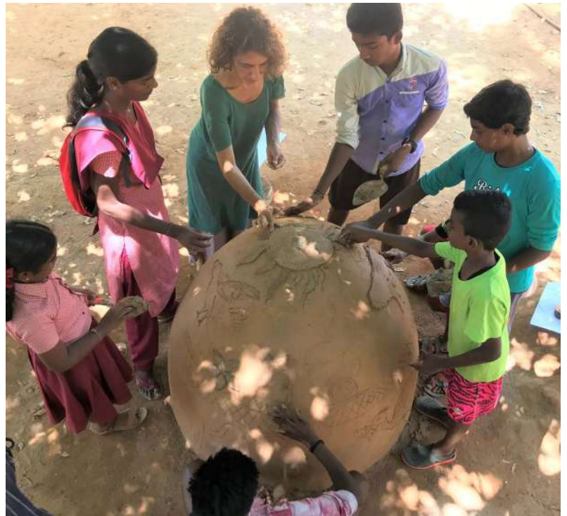
Students plastering and decorating the exterior of the dome
