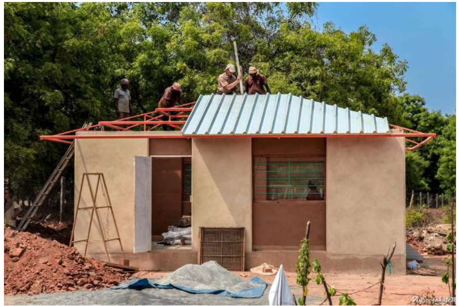
The roof going onto the social space at Anitya
