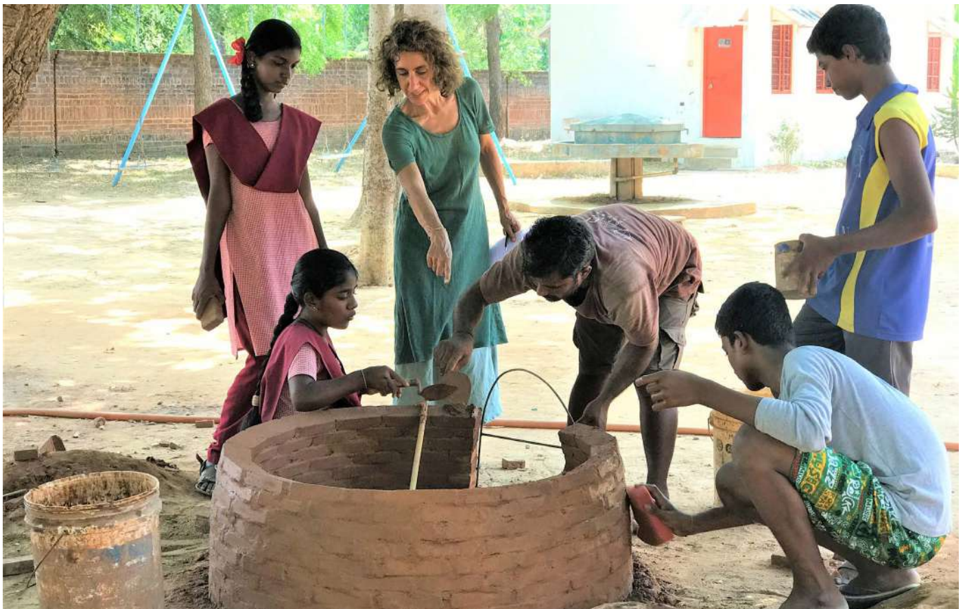
Students working on the dome at Udavi School
