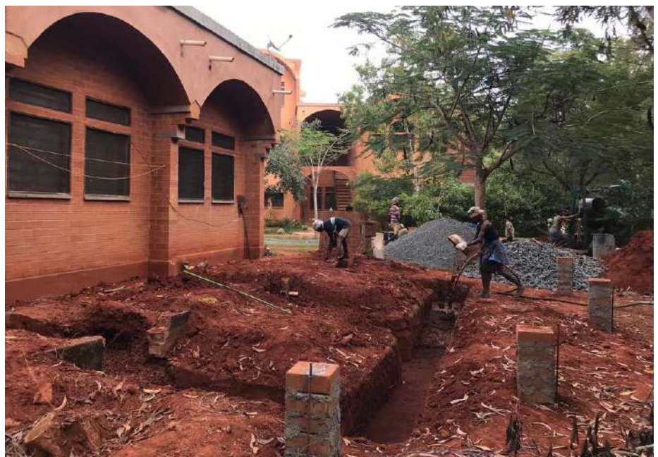
Construction beginning on Jayaraman's extension
