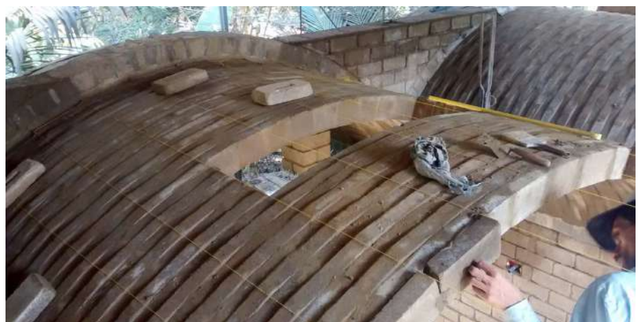
Vault construction in progress
