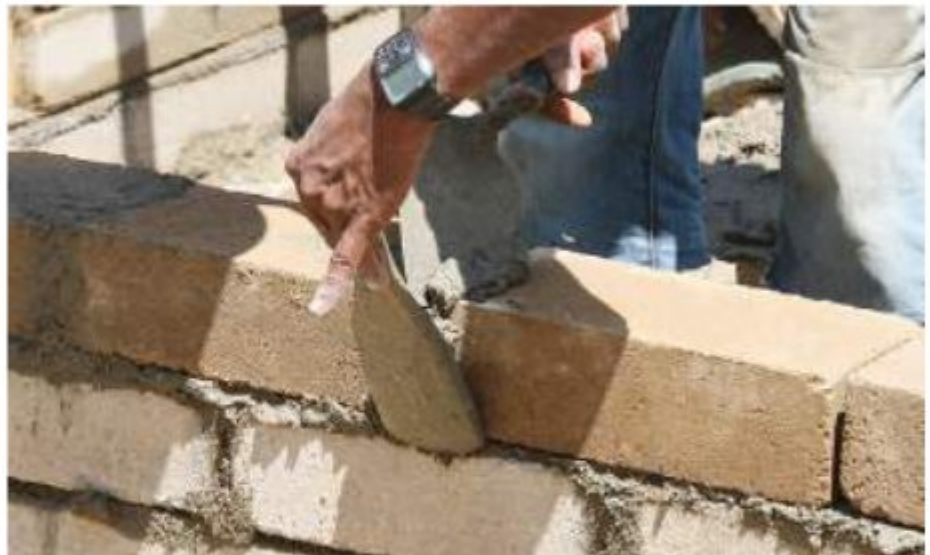
Ongoing work for the HfHSL "Homes Not Houses" project.
