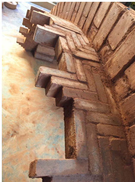
Mostafa working on a Persian herringbone bond pattern
