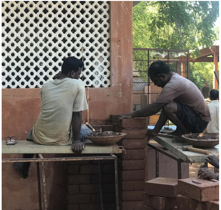
Sambasivam and Mani working on Priya's extension
