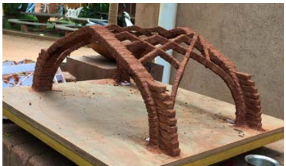
Behnaz and Pouya finishing up the formwork; a view of the “Karbandi” dome with the formwork still in place; the completed free-standing “Karbandi” dome
