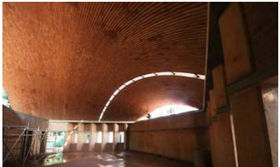
Completed earthen conical vault of the Sharanam Conference Hall
