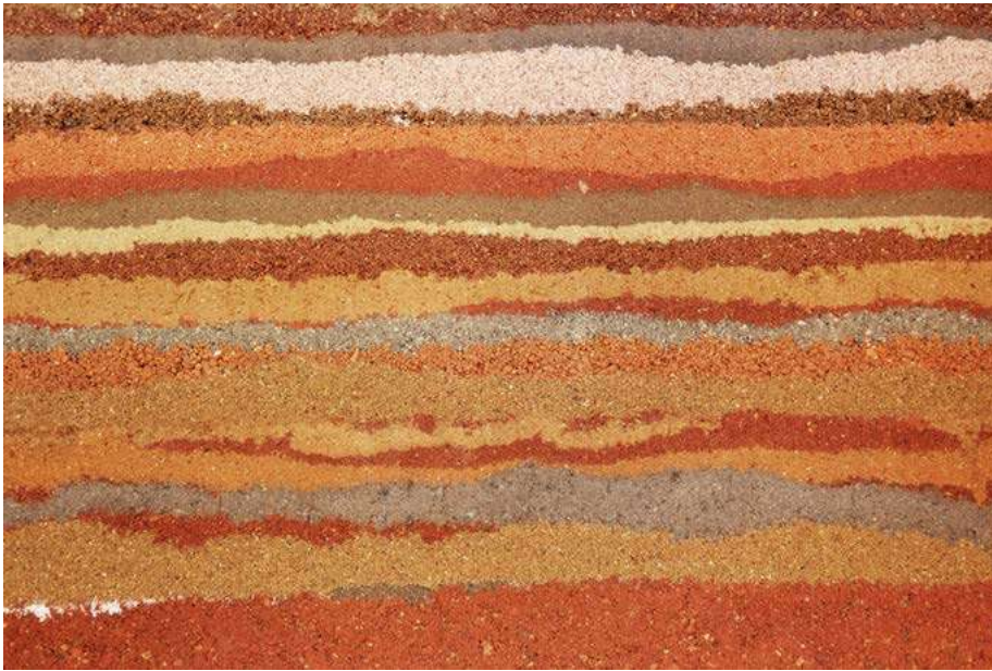
A close up of the finished Rammed Earth Stele
