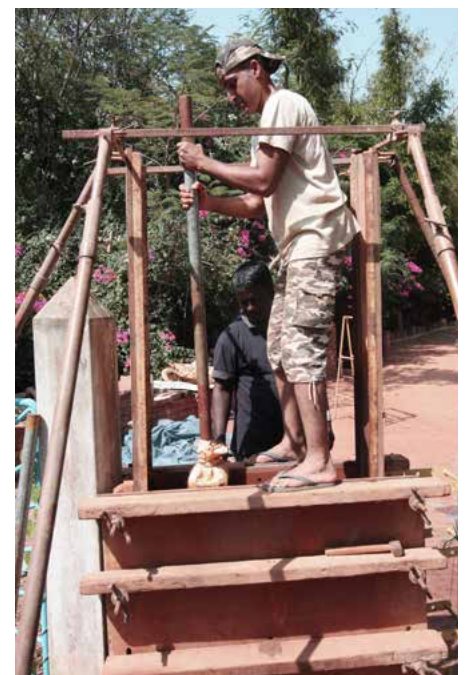
Ramming a wall within a formwork
