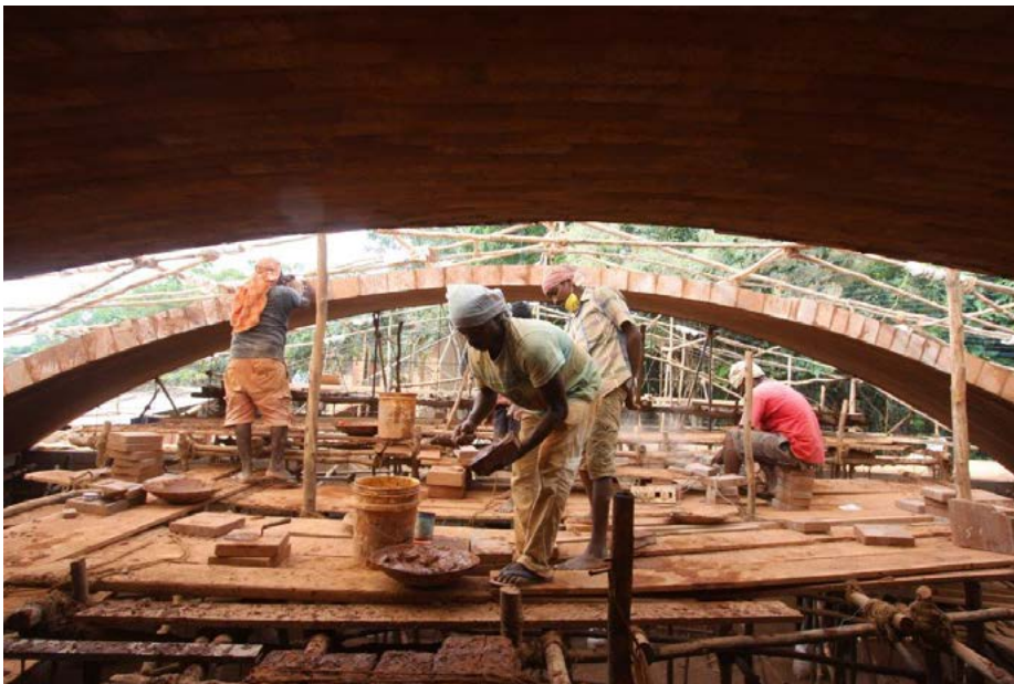
Working on the 15 m conical vault at Sharanam
