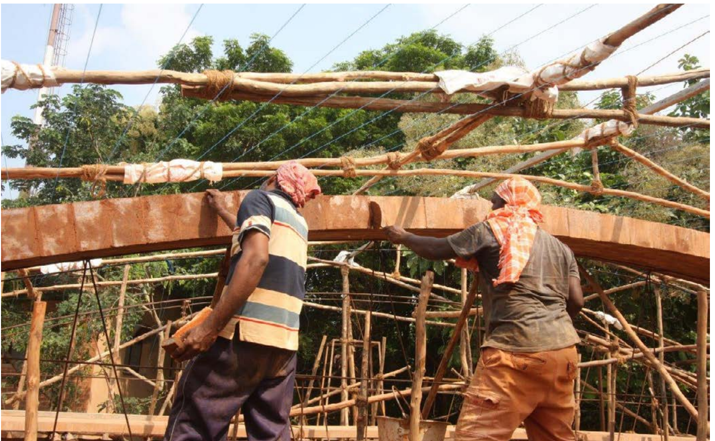
First courses of CSEB at the widest span of the vault
