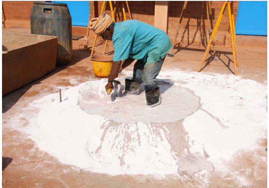
Mixing water into a lime stabilized earth plaster
