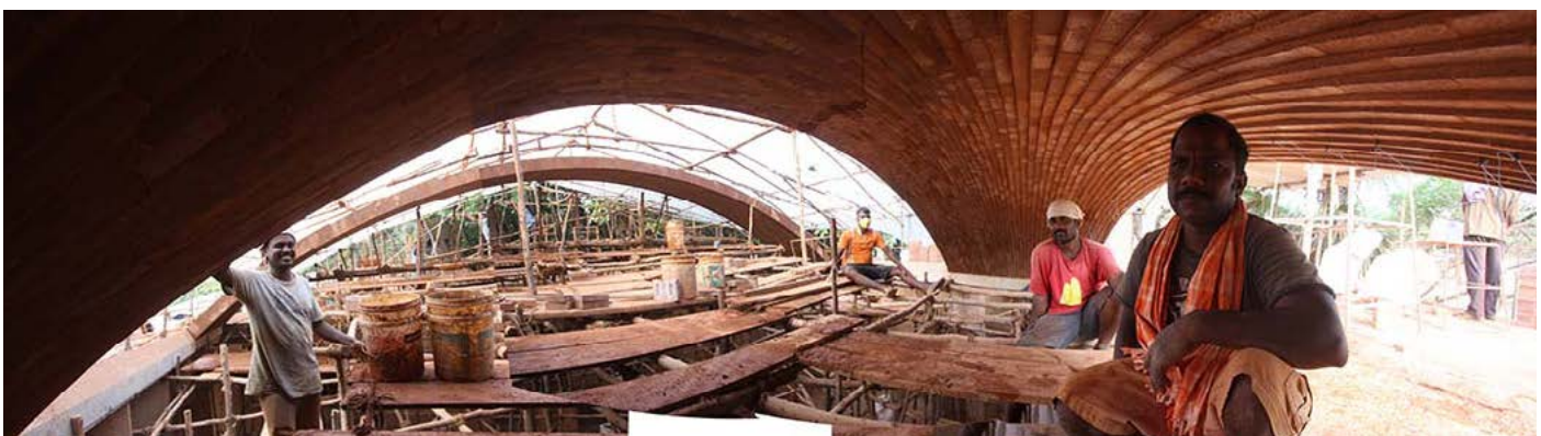
Head masons at work laying the successive courses of CSEB
