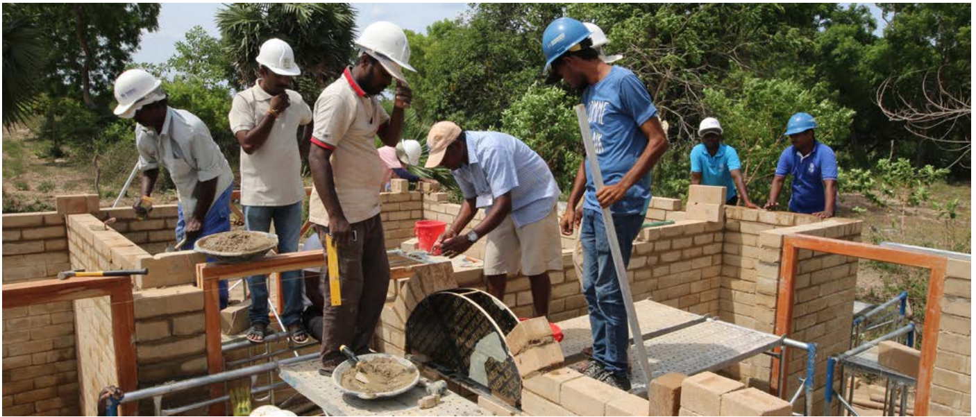
Ayyappan teaching HfHSL trainees and masons how to build an arch
