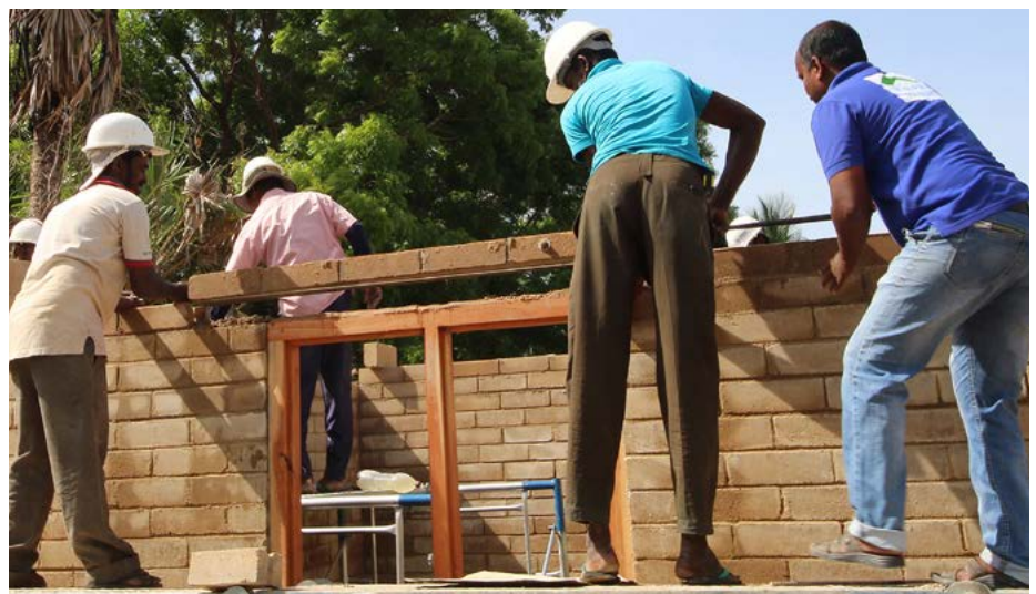
Trainees laying composite lintels
