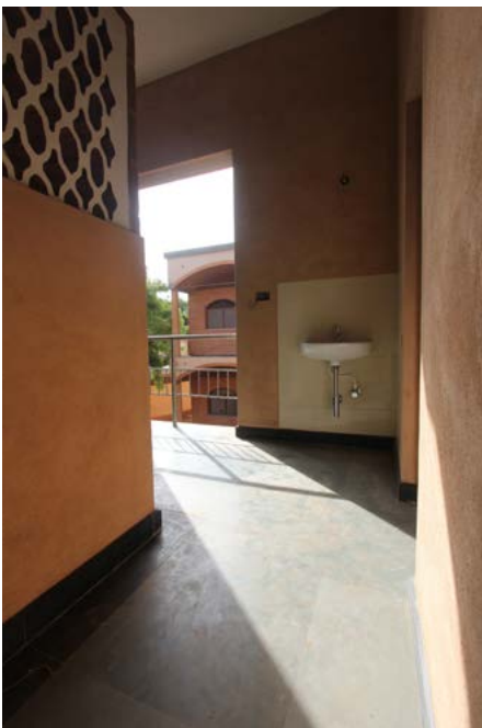
Views of the double story residential units, with CSEB walls and vaulting, jaali ventilation, lime plaster, and stone flooring
