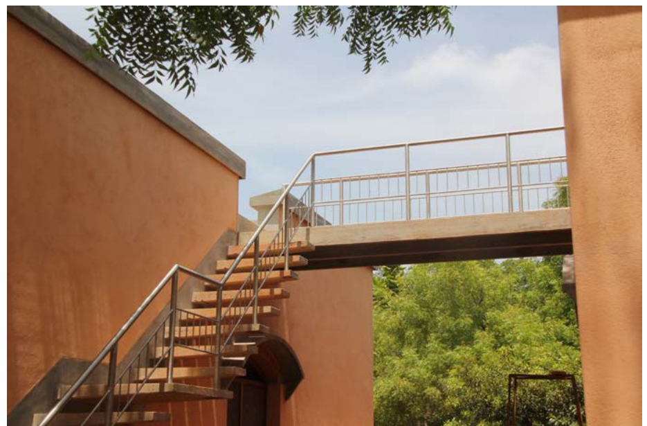
Single story units flanking the PEC road, with interconnected roof terraces
