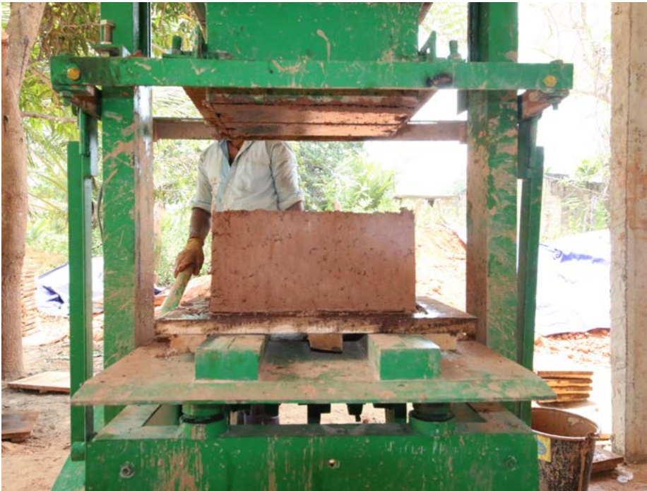
Earth Concrete Block production starts in Sri Lanka
