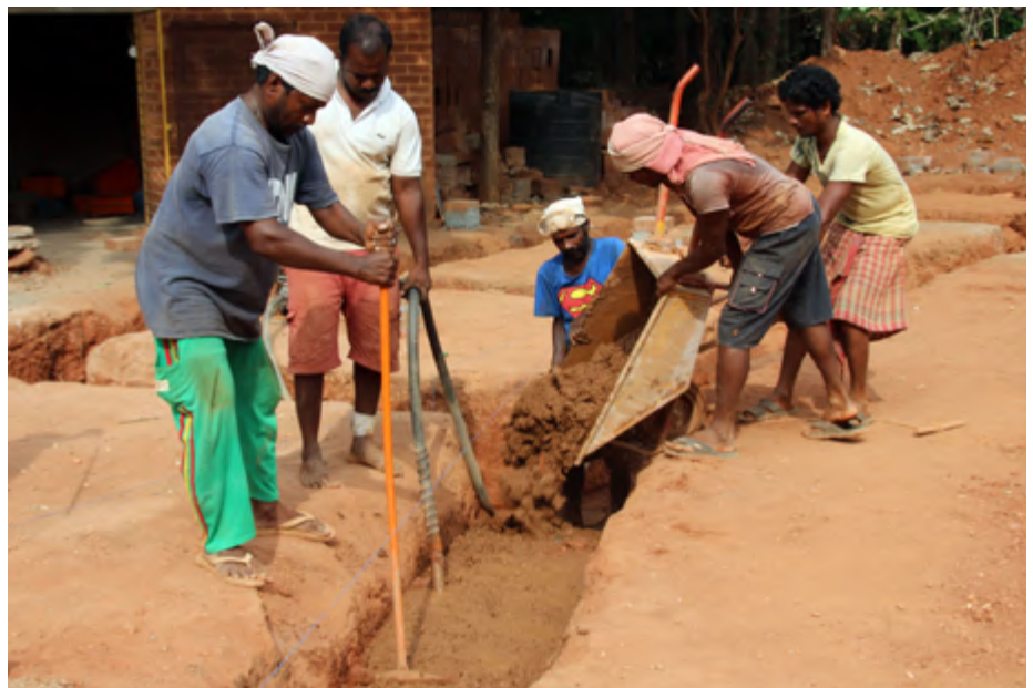
Spreading and vibrating the PEC for the conference hall foundations
