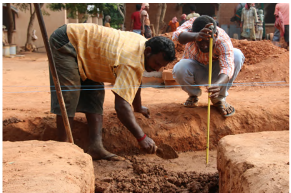
Controlling the levels at the top of the foundation
