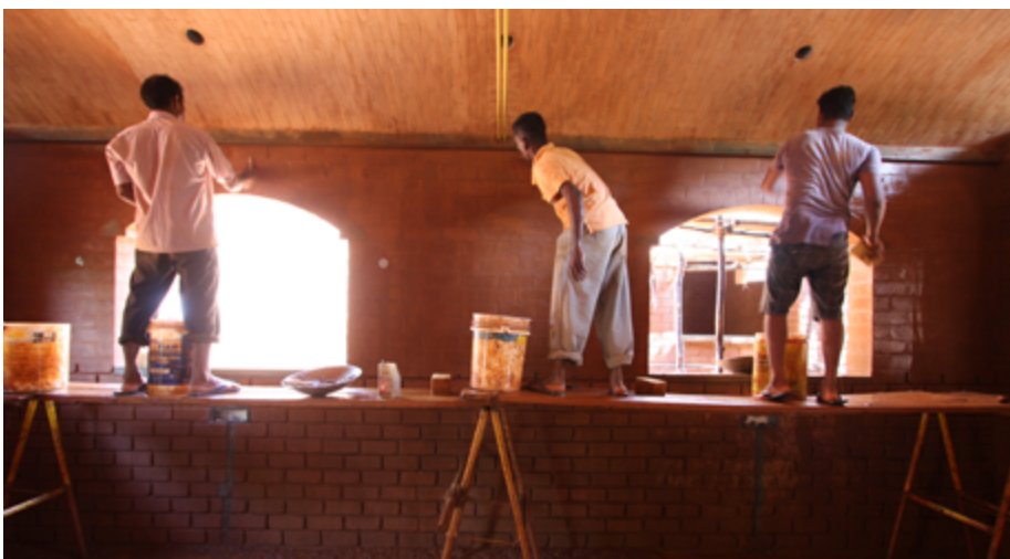
Interior finishes at Sharanam
