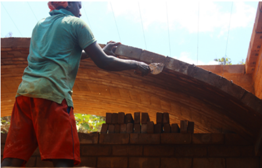
Vault construction progressing on the Sharanam Phase II buildings
