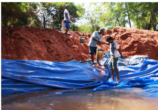
Monsoon rain collecting in the excavation pit
