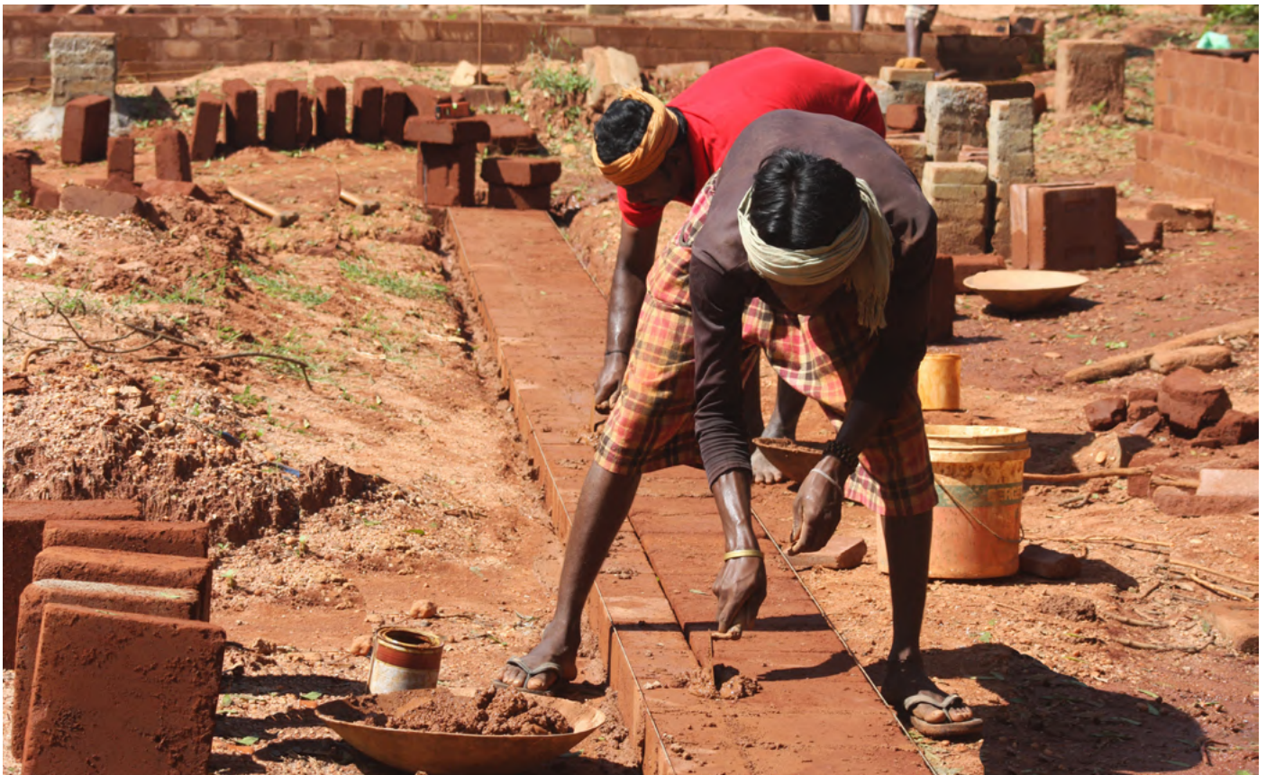
Masons working on the basement of the single-story buildings at Sharanam
