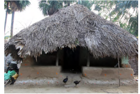
A well-built cob house with a keet roof
