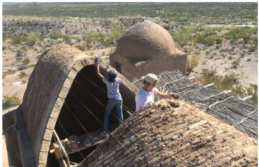
Alex Williams and Beatrice Denham rebuilding the adobe nubian vault
