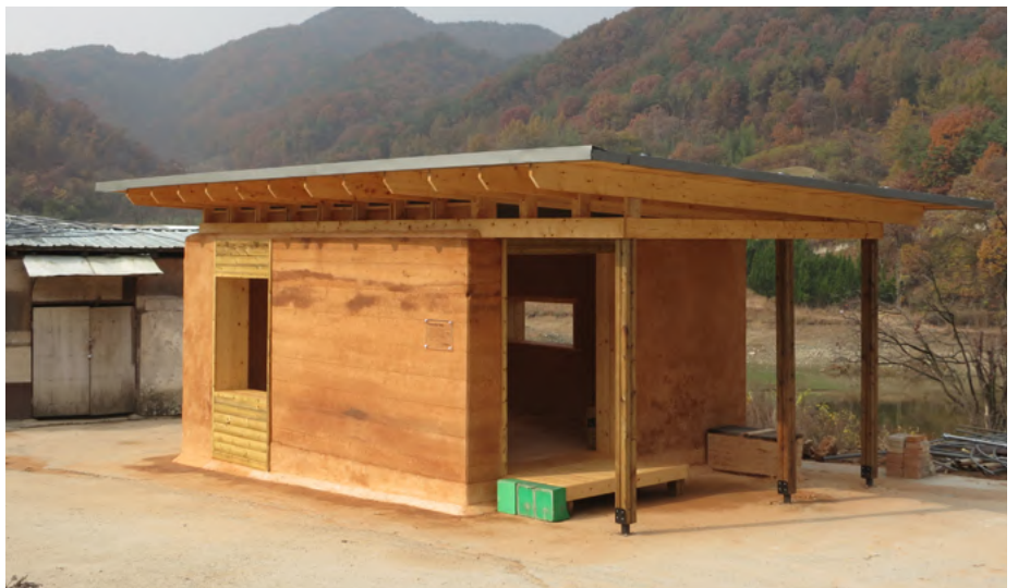
A small building constructed by students during a recent training course
