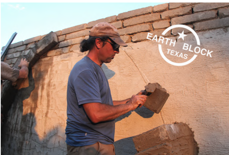
Arch and "Free-Spanning" vault construction with CSEB and earth mortars
