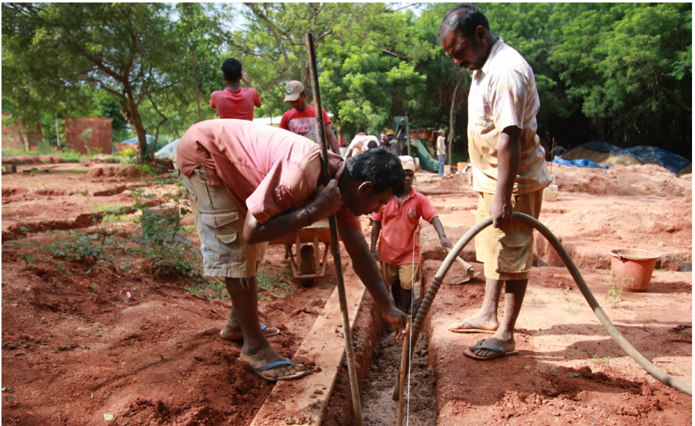
Casting Poured Earth Concrete foundations at Sharanam
