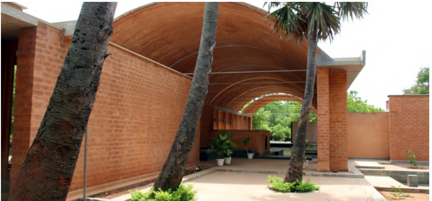
Exterior view of the Phase I main hall
