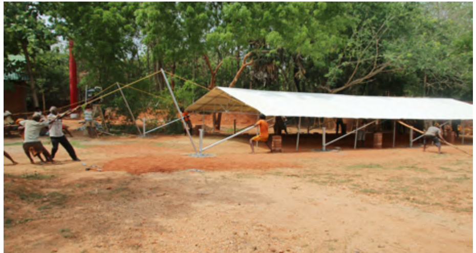
Erecting the blockyard shed
