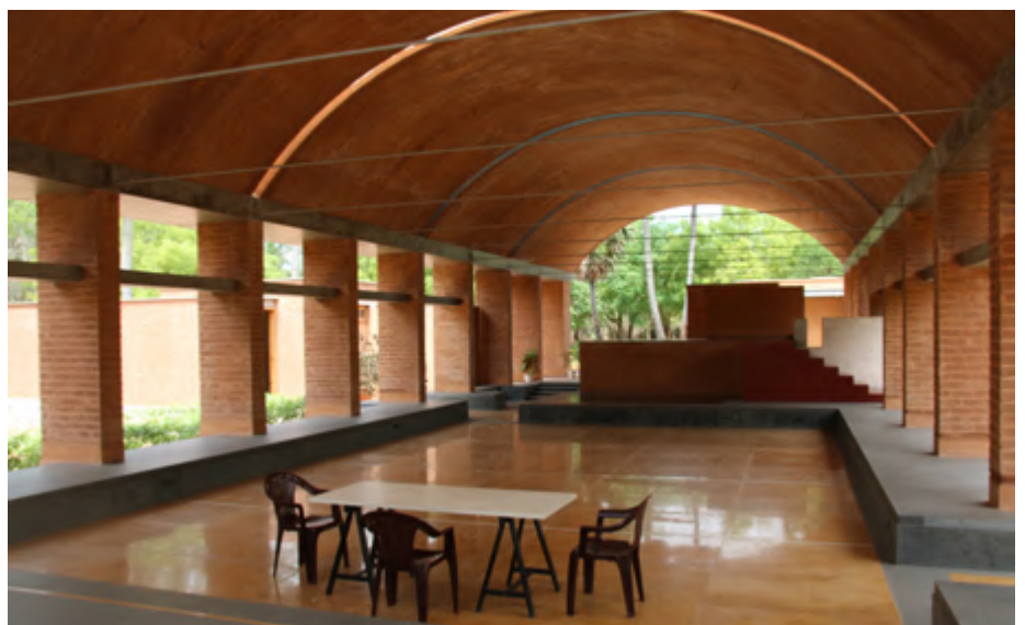
Interior of the CSEB vault spanning 9.5 meters
