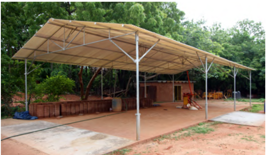
Finished blockyard shed with blocks curing
