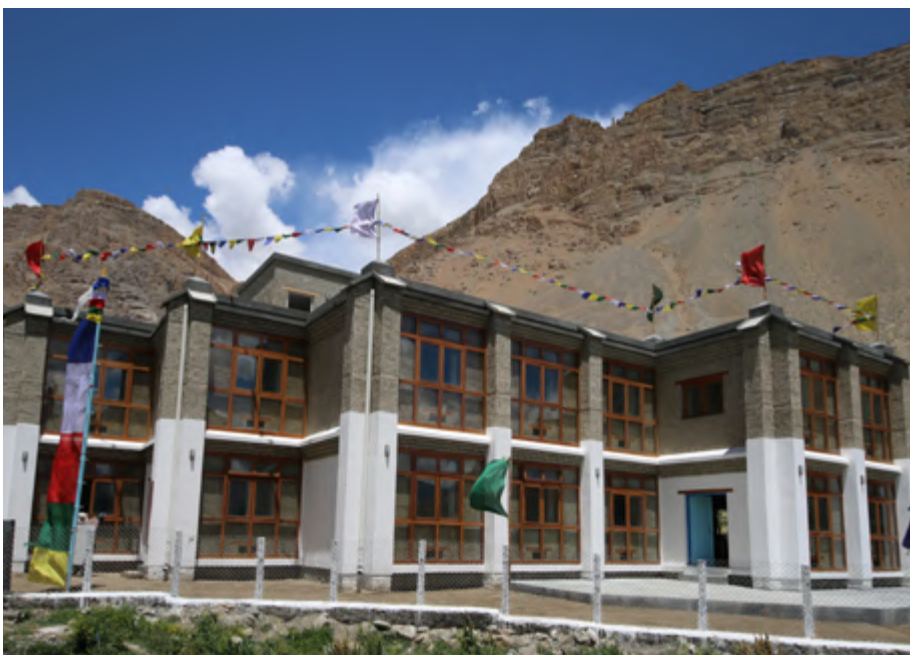
Completed exterior of the Kaza Community Centre
