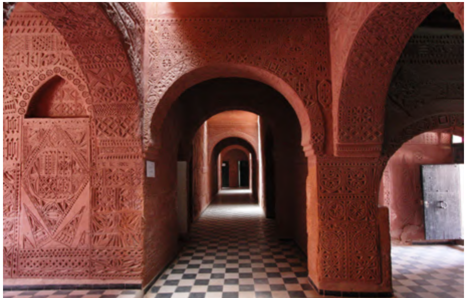
Oasis Rouge in Timimoun, made from adobe and intricate earthen plasterwork
