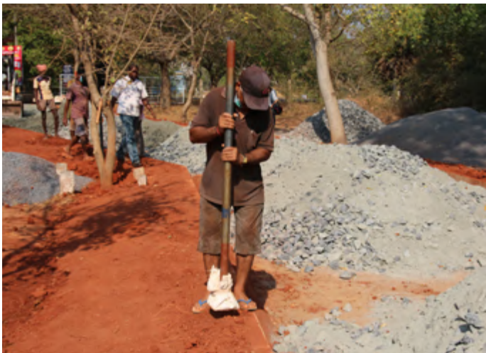
Tamping the raw red earth slopes up to the roadway
