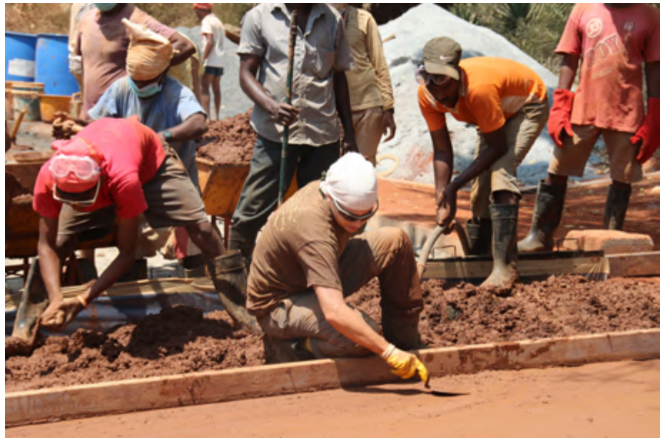
Filling gaps in the wearing course
