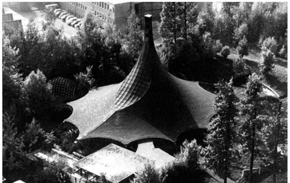
ILEK tent structure, originally erected as a prototype to test the construction and assembly of the German Pavilion for the World Expo 1967 in Montreal. (photos: ILEK)
