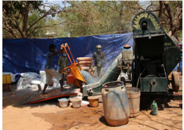
Filling the cement mixer with the PEC
