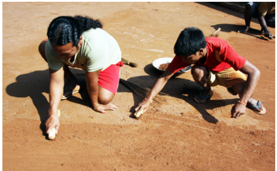
Giving a rough finish to the road with wire brushes
