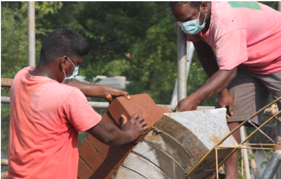
Work on the arches of the Sri Vast Ashram Entrance Building
