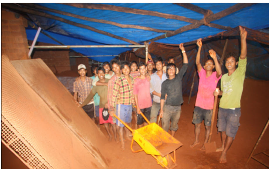
Sieving soil under tarps to protect from the monsoon rains
