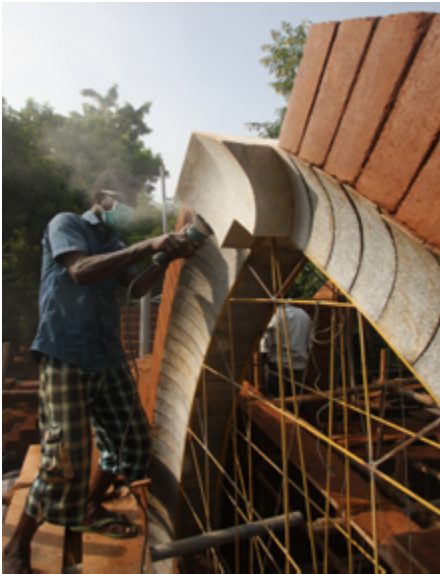
Grinding the keystones for the arches
