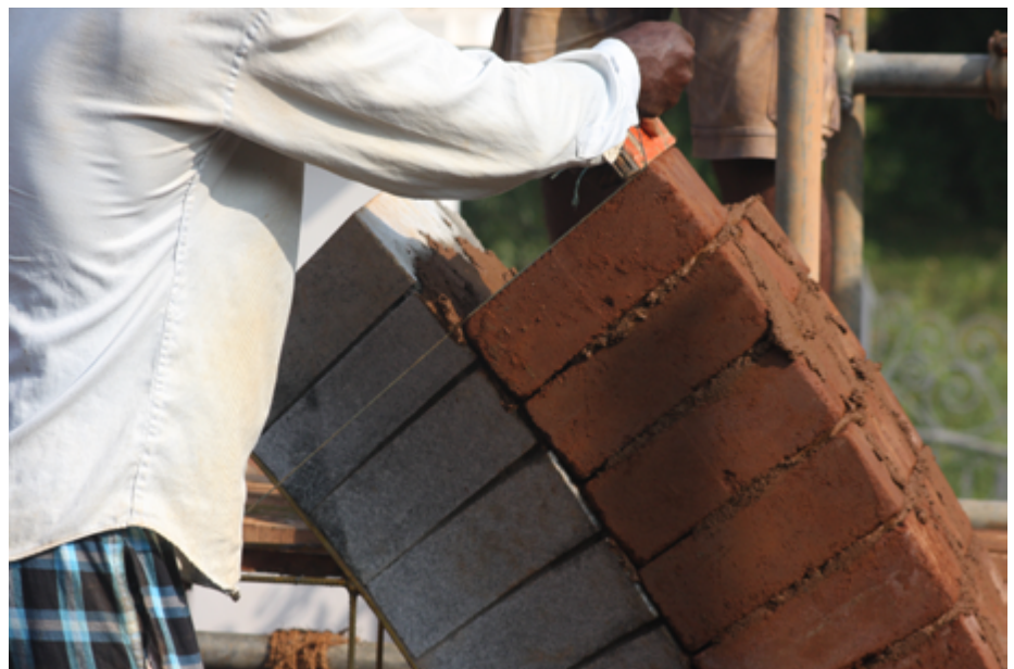
Laying CSEB over the stone arches of the Reception Building
