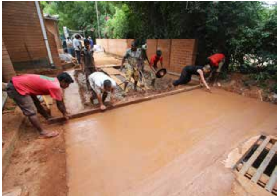
Screeding the road and filling in any holes with trowels
