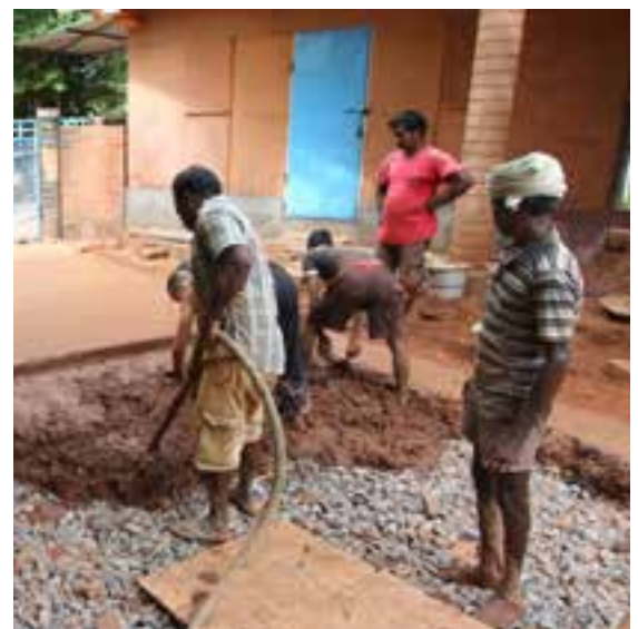
Applying and vibrating the earth concrete
