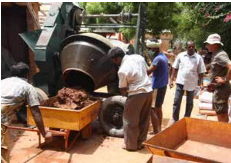
Satprem and Ayyappan overseeing the mixing of the earth concrete
