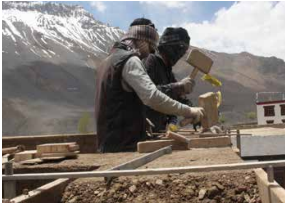
Ramming the first floor walls with mallets
