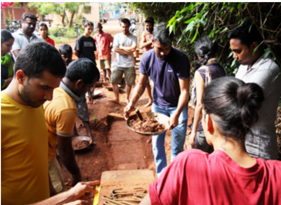
Trainees working on a CSEB wall
