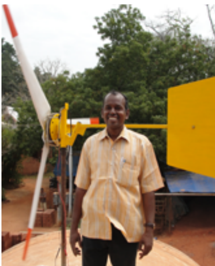
Ayyappan with his 5 kW wind turbine
