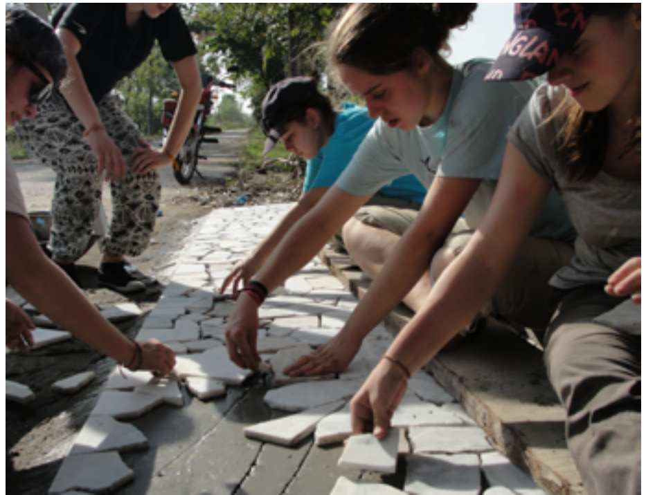
Belgian volunteers laying marble tiles for the patio
