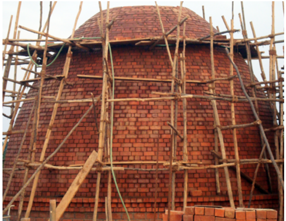
The dome in the final stage of construction
