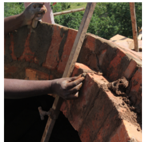
Mani working on the intrados of the dome
