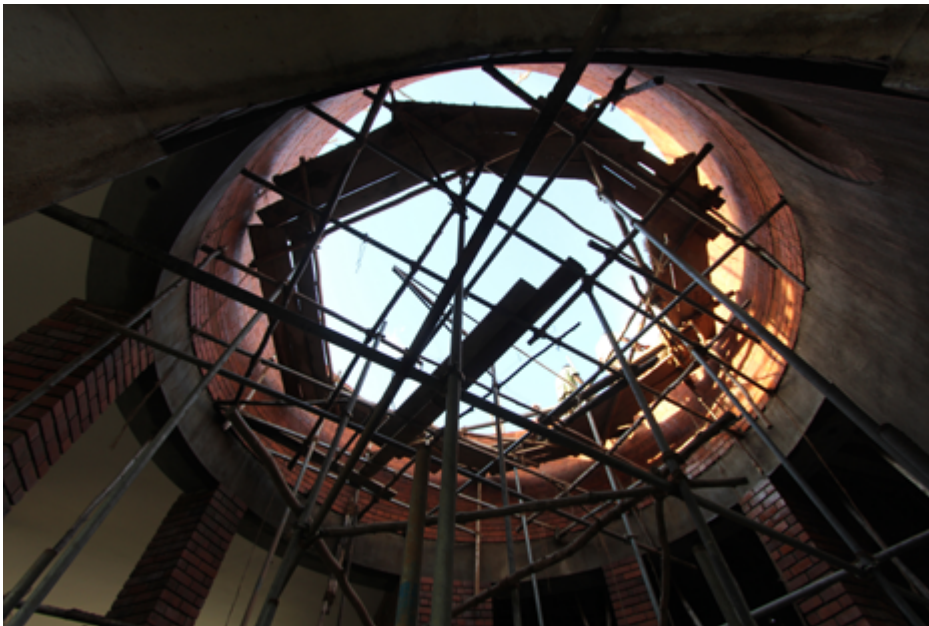
Scaffoldings inside the dome at Sri Vast Ashram
