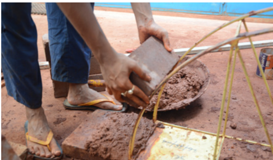
AVD Masonry in action
