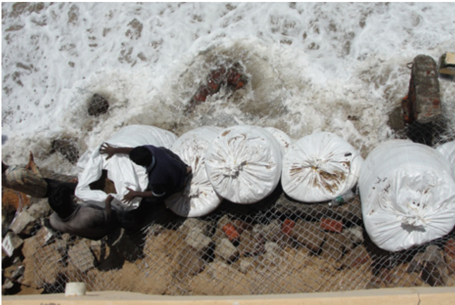
Earth Institute workers fighting the sea to fill sandbags at Repos, Auroville
