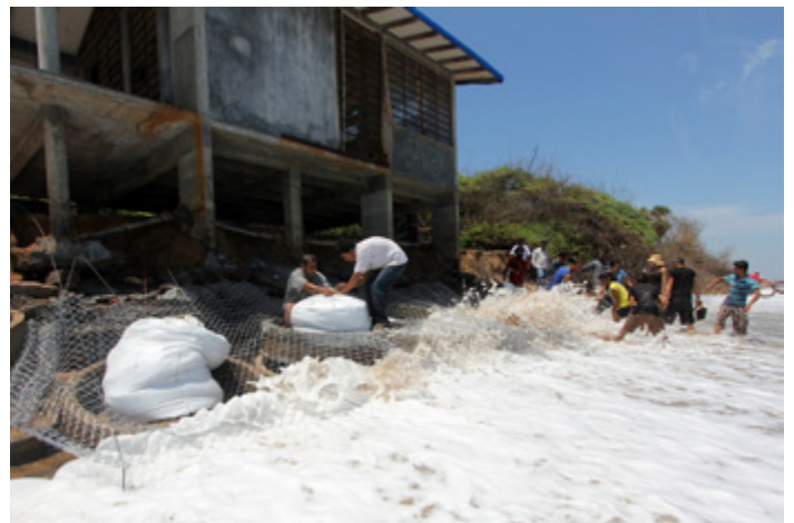
Volunteers working to fill sandbags in the surf
