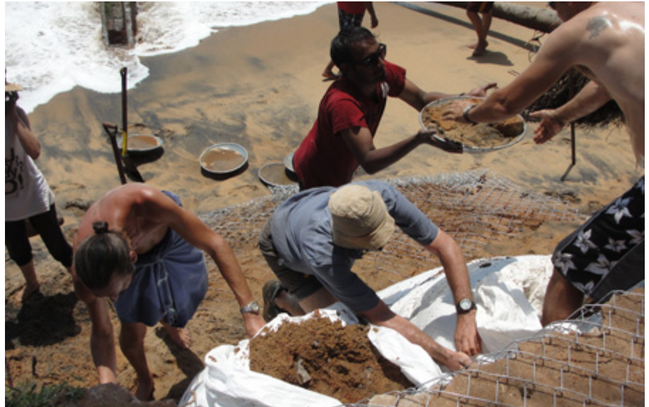
Filling sandbags to prevent eroding under the guest house's foundations
