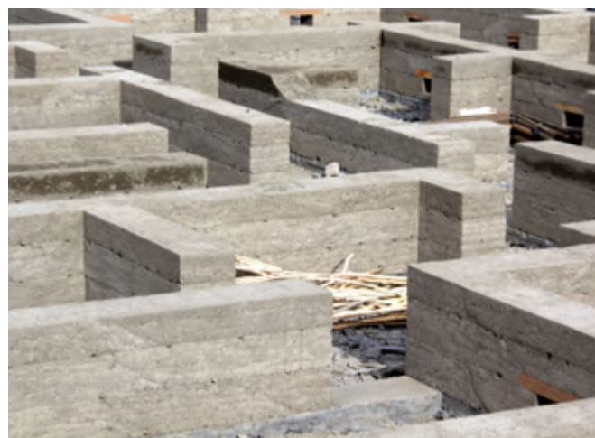
Rammed earth walls built up to the sill level
