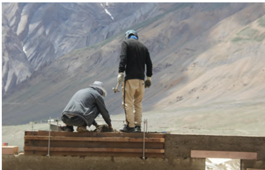
Rammed earth with the vernacular “wet” technique of Spiti Valley
