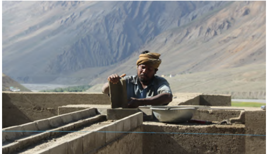
Crew member of the Kaza Community Center construction laying CSEB
