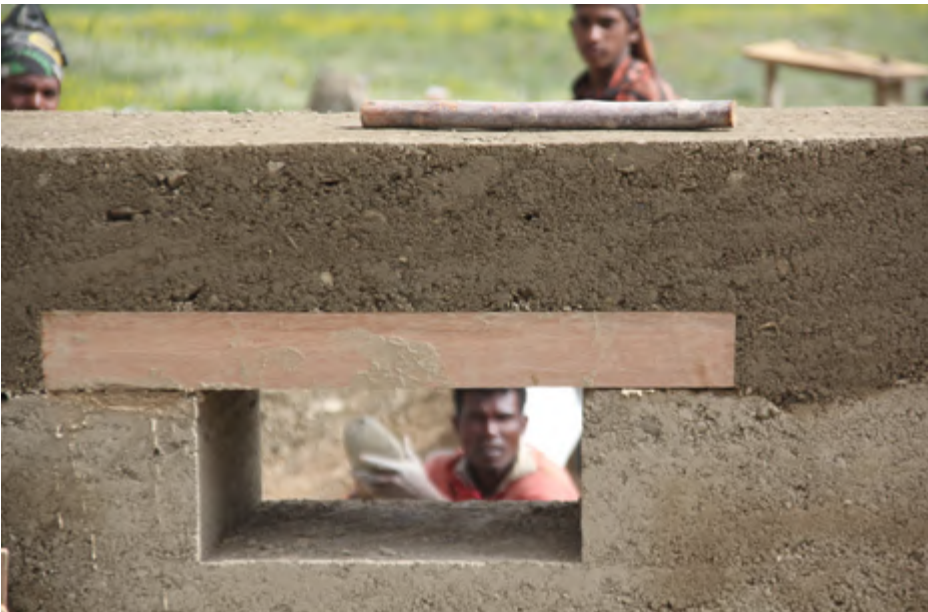
Eco-Community Center construction in Kaza, Spiti Valley, India
