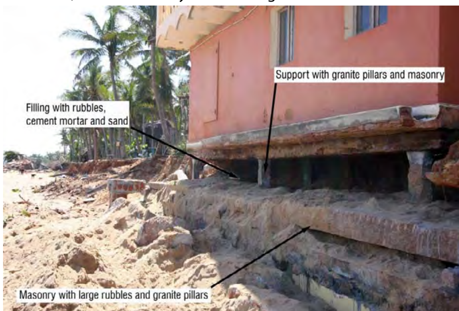
Reinforcement to the foundation done by the AVEI
