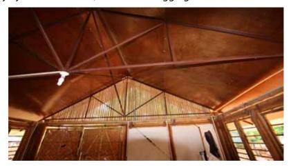
Steel trusses & ply-wood ceiling
