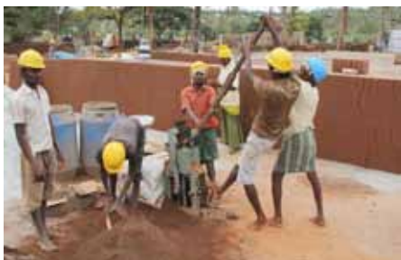
Block Production at Malhar
