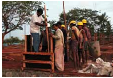
Rammed Earth Wall Training
