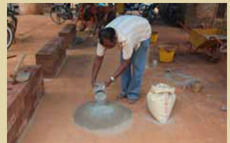
Mixing the Grout
