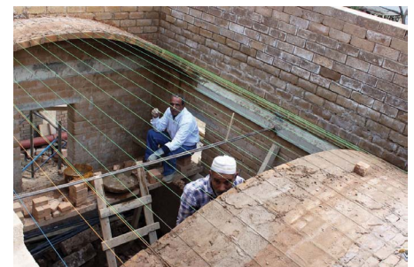
Building a segmental vault
