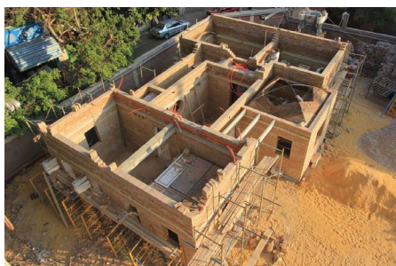
Pointed cloister dome in progress
