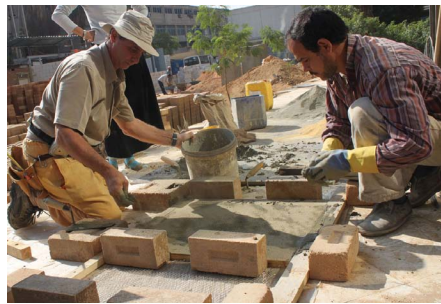
Casting ferrocement slabs
