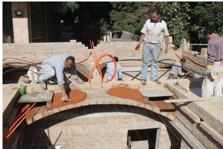
Cavities for the flooring of the vault
