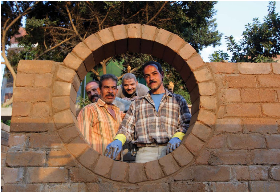
Finished round arch in Egypt - December 2011
